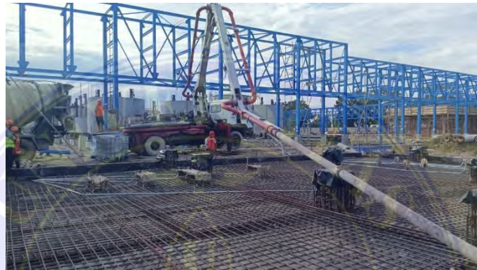
Gambar 3.7. Concrete Pump Truck (Dokumentasi Proyek, 2025)
