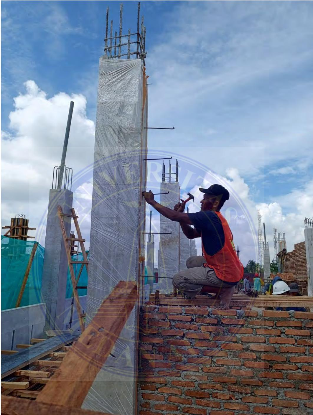
**Gambar perawatan beton kolom**
