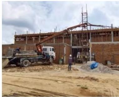
Gambar 5. *Concrete Pump truck* (Dokumentasi Proyek, 2025)
