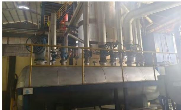
**Gambar 3.46 Back Pressure Vessel**
