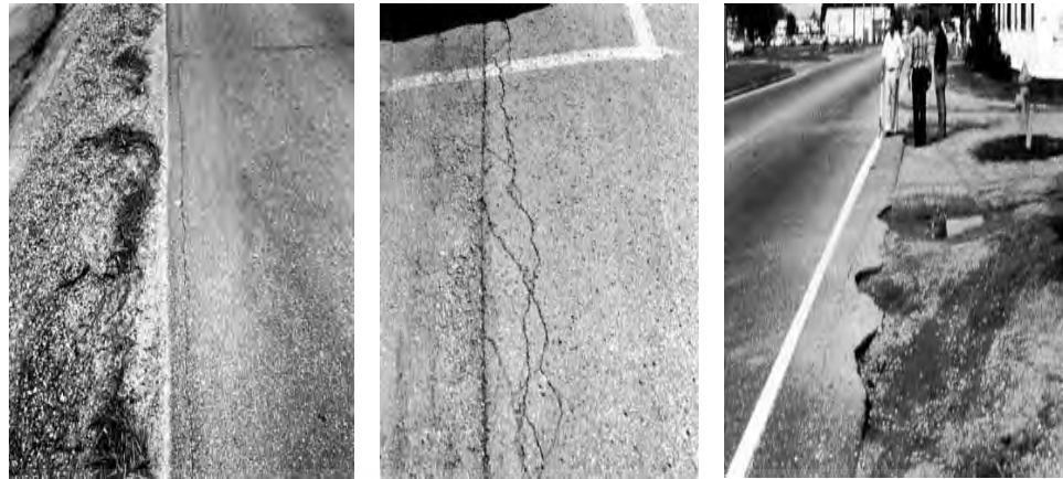
(a) Low (L) (b) Medium (M) (c) High (H) Gambar 2 Retak pinggir ( Edge Cracking ) (ASTM International, 2018)
