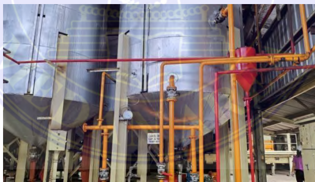
Gambar 3. 25 Clean Oil Tank
