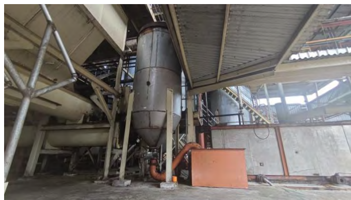
Gambar 3. 19 Sand Trap Tank
