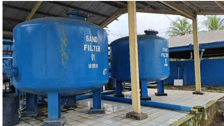
Gambar 3. 54 Sand Filter
