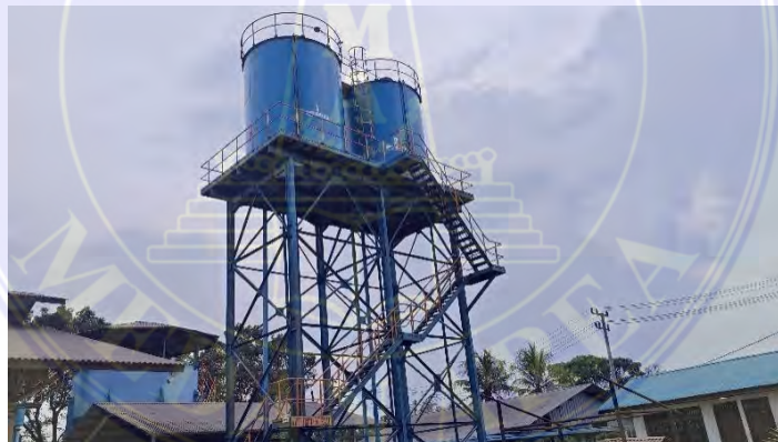
Gambar 3. 55 Water Tower Tank
