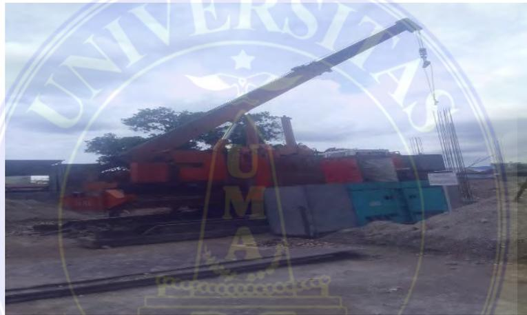
Gambar 3. 1 HSPD (*Hydraulic Static Pile Drive*)
