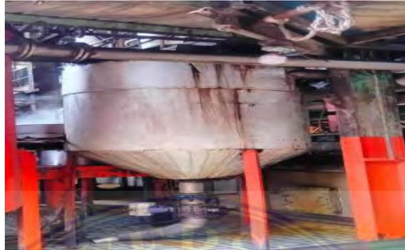
**Gambar 3. 31 Sand Trap Tank**
