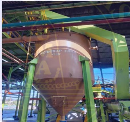
**Gambar 3.5. Sand Trap Tank**
