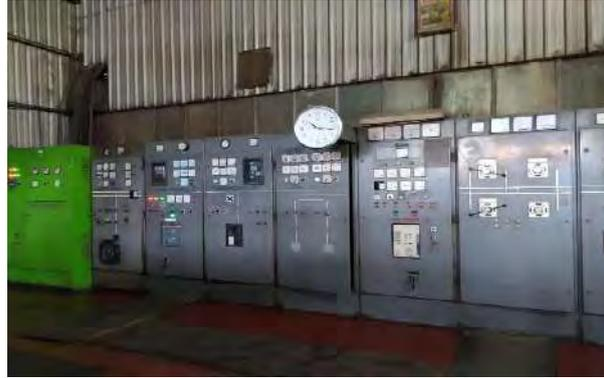
Gambar 3.57 Main Switch Distribution Board ( Panel Kontrol Utama )
