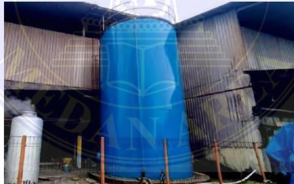
Gambar 3.64 Feed Water Tank
