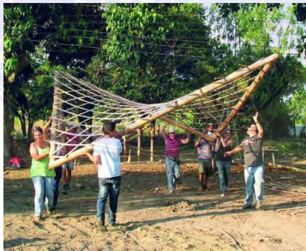
Gambar 2. 2 penerapan hyperbolic paraboloid
