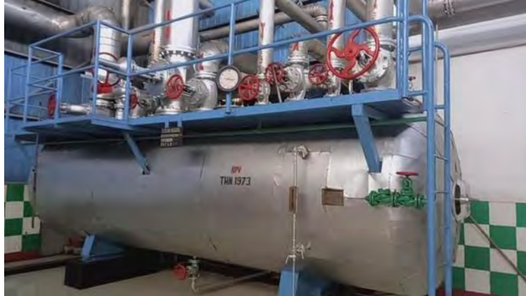
Gambar 3. 46. Back Pressure Vessel (BPV)
