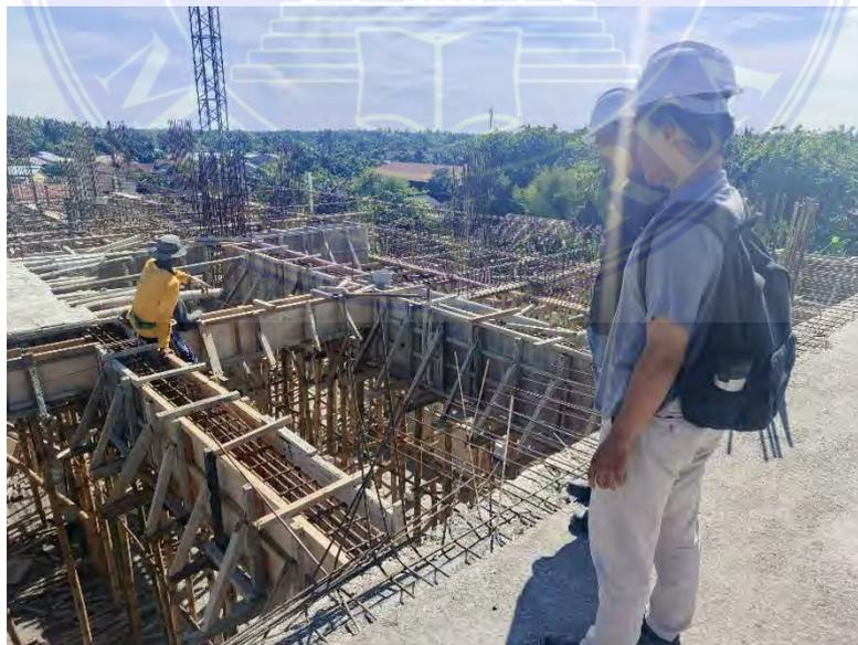
*Gambar 3 3 Bekisting (Formwork)*
