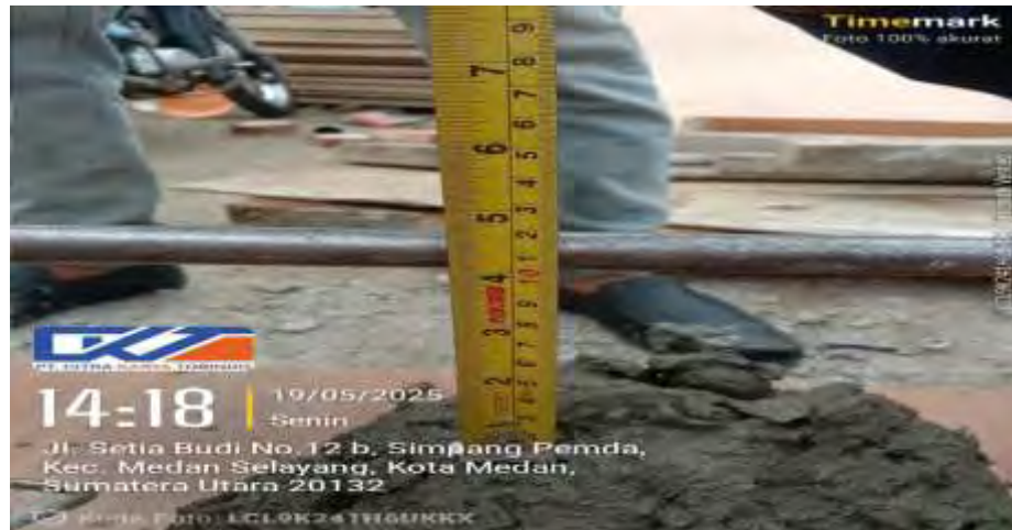
Slump Test Beton Balok
