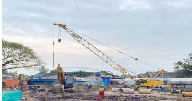
Gambar 9 Tower crane (Dokumentasi,2025)
