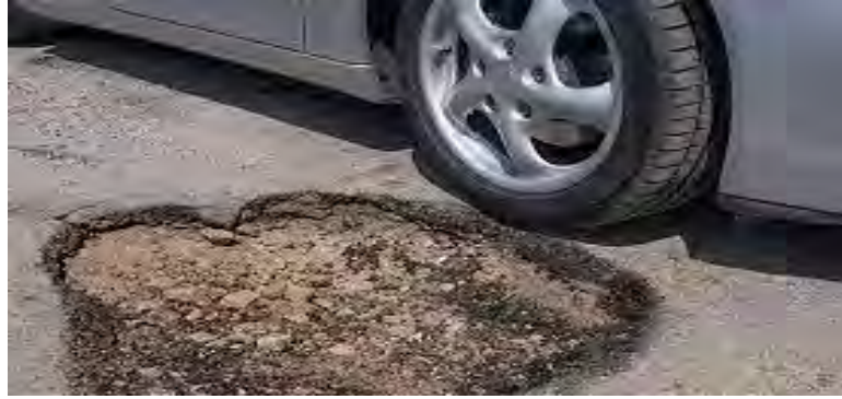
Gambar 11. Lubang ( Potholes )
