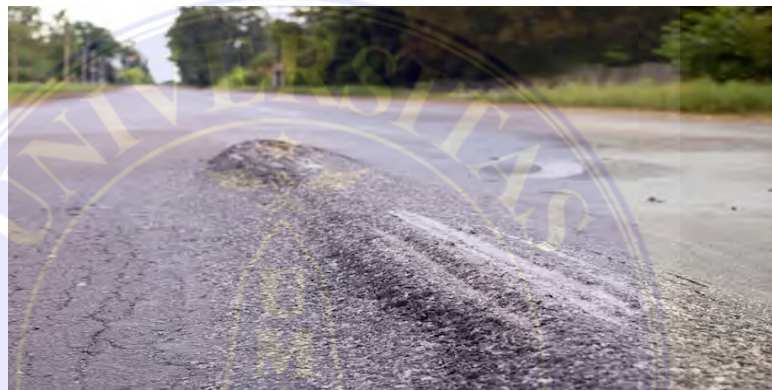
Gambar 9. Retak Sungkur ( Rutting )
