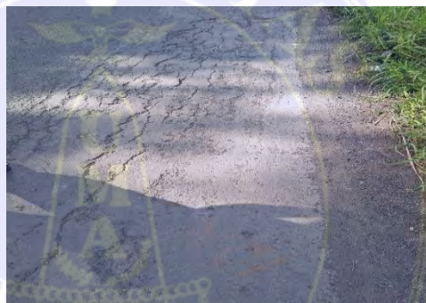
Gambar 8 Retak Sambungan Bahu Jalan (Shahin, 1994)
