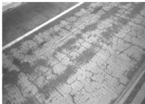
Gambar 12 Retak Susut (Shahin, 1994)
