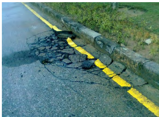
Gambar 7 Retak Pinggir (Shahin, 1994)
