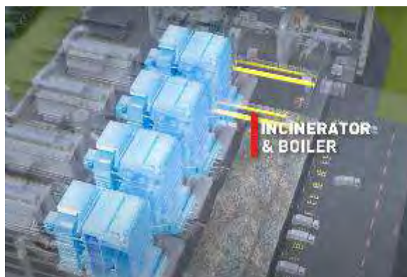
Gambar 2. 27 Incinerator & Boiler TuasOne WtE Plant
