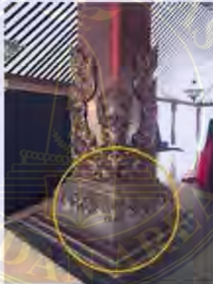
Gambar 2. 15 Umpak Pendopo
