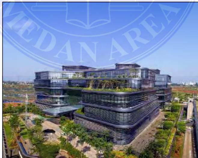
Gambar 2.19 BSD Green Office Park Sumber: www.archdaily.com
