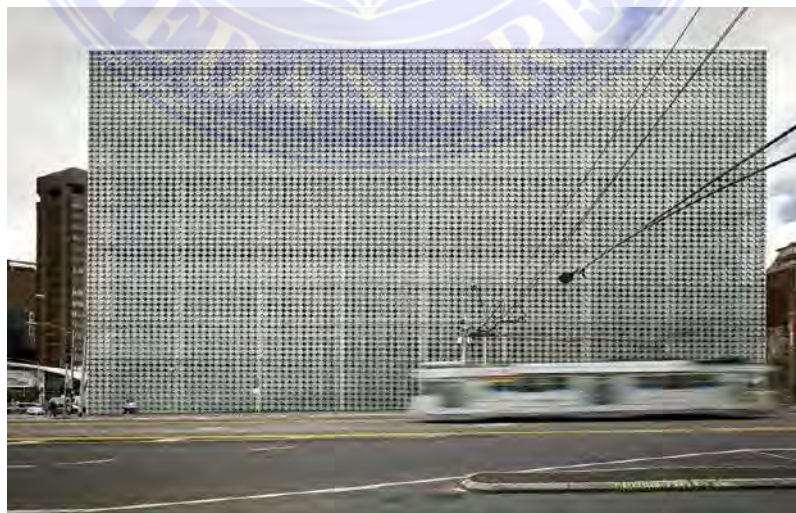
Gambar 2.10 Fasad RMIT Design Hub Sumber: www.architecturalrecord.com
