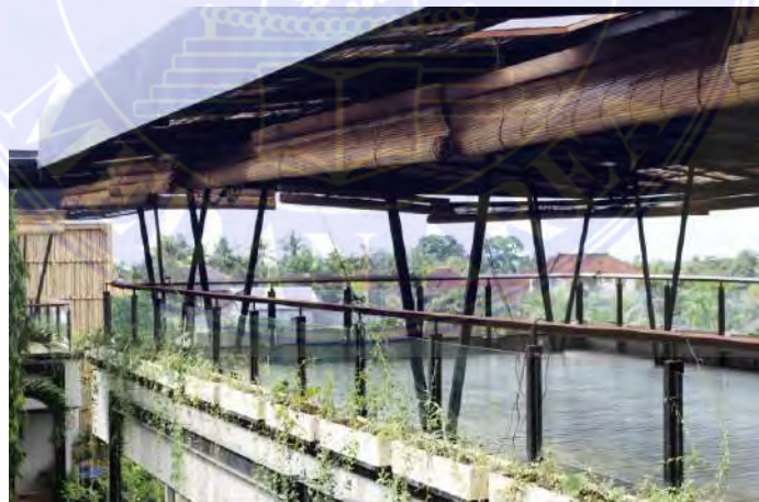
Gambar 2.14 Area Rooftop/Area Coworking space
