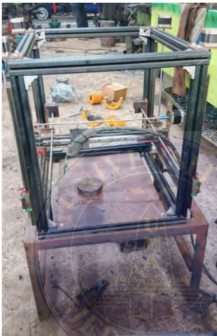
Gambar proses perakitan frame mesin 3d printer welding
