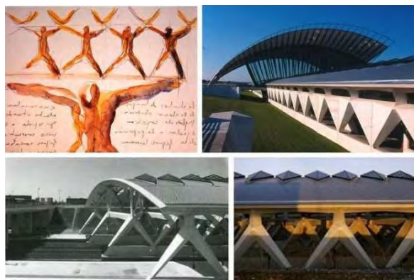
Gambar II.8. Bangunan Saint Exupéry Airport Railway Station, Lyon – Satolas
