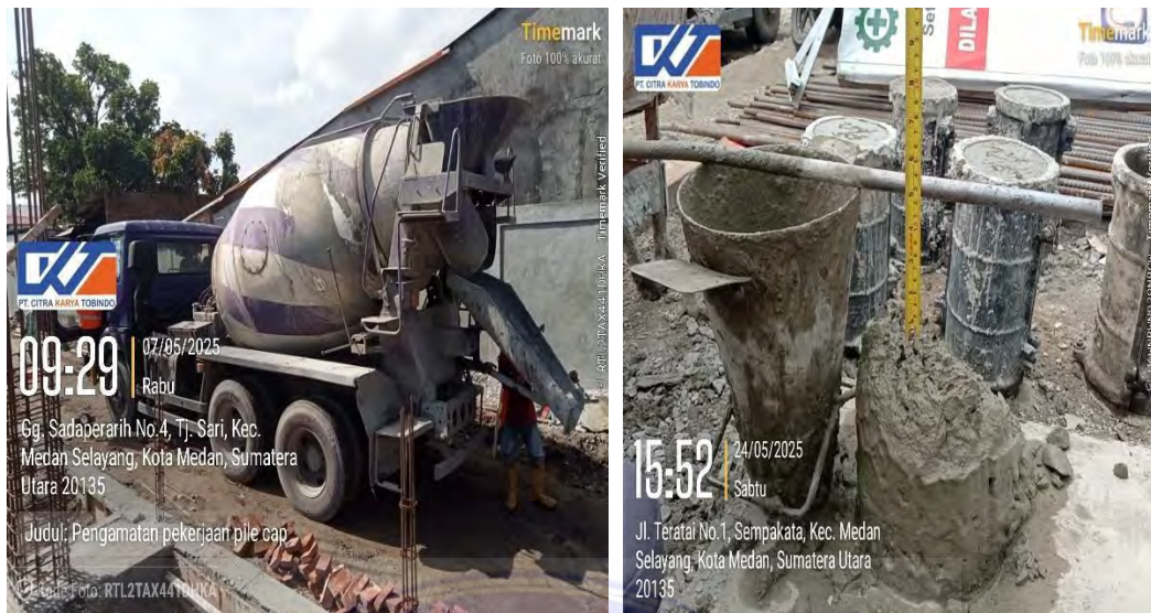
Gambar Uji slump beton
