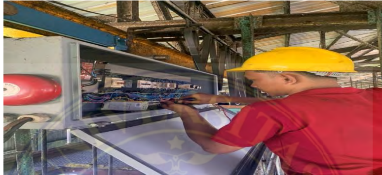
Gambar 4.6: Pemasangan Relay Voltage
