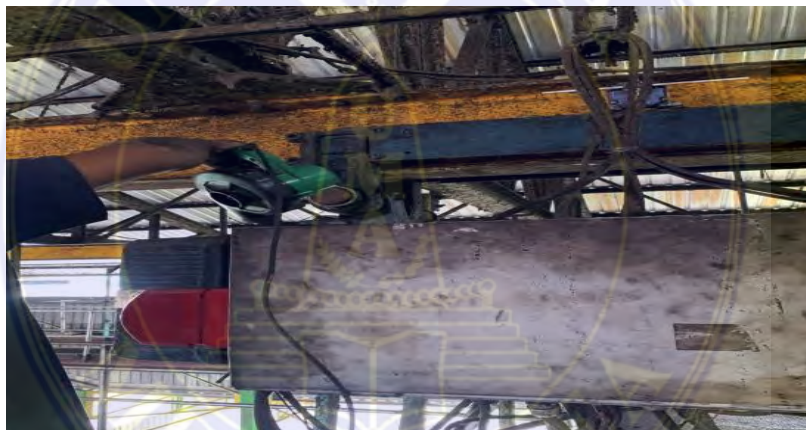
Gambar 4.2 Pembersihan Panel Kontrol Hoisting Crane
