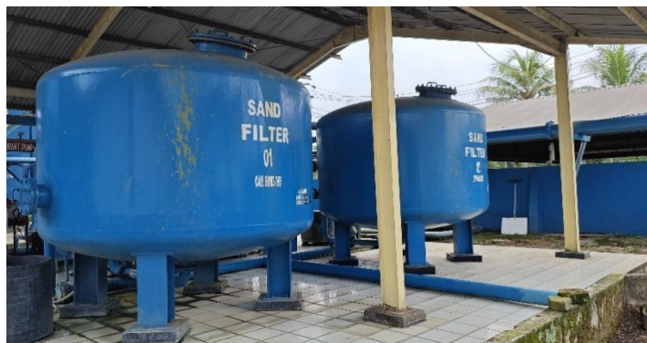
Gambar 3. 58 Sand Filter
