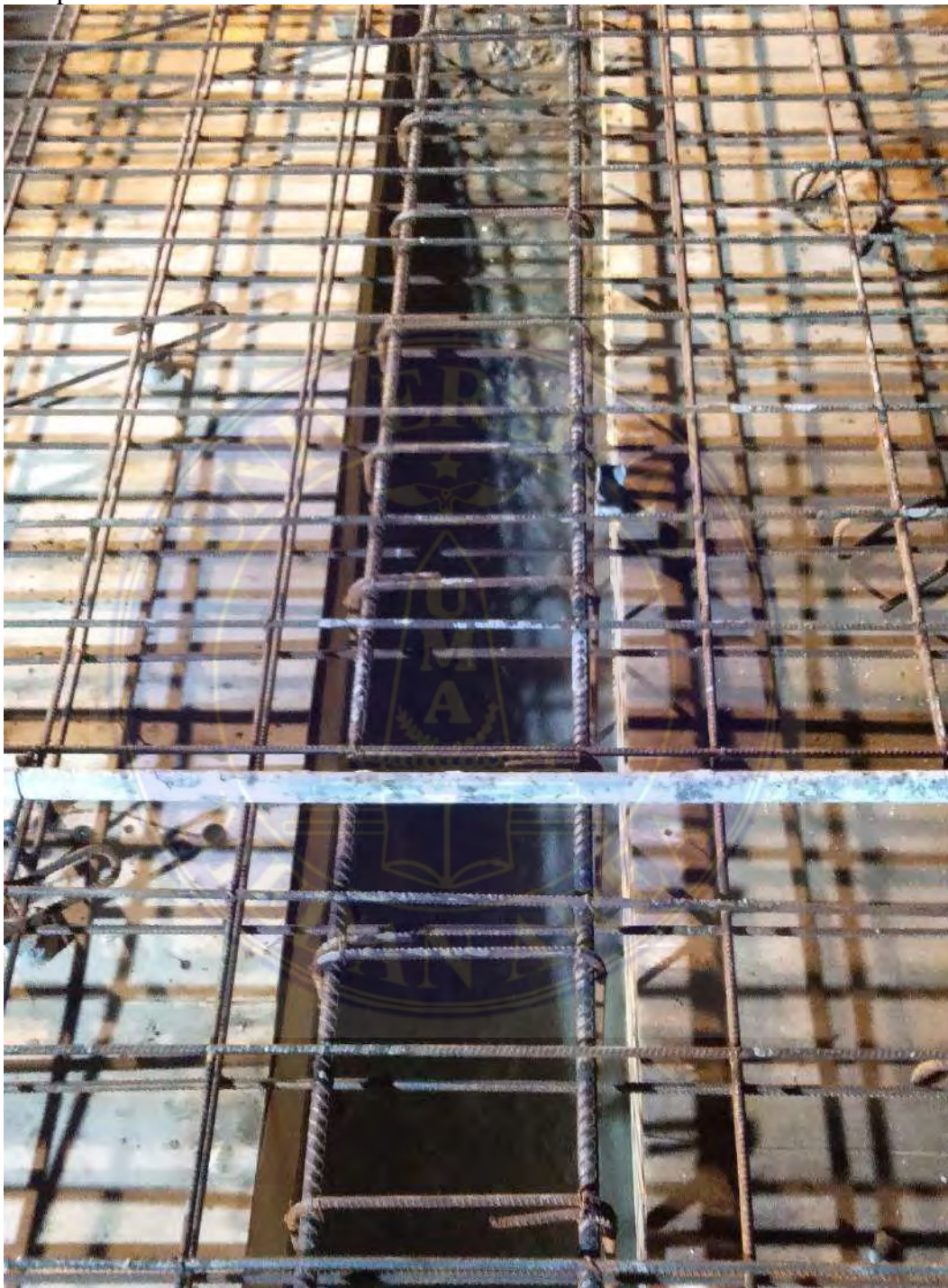
Lampiran 1. Gambar detail balok
