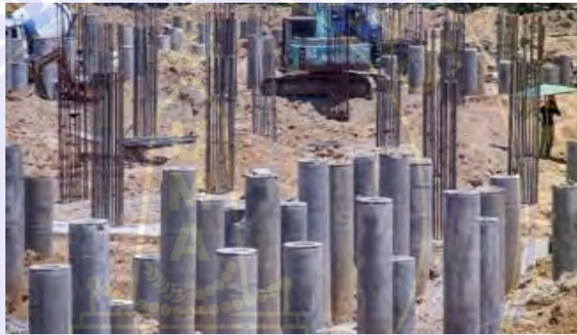
Gambar 7. Pondasi Tiang Pancang (Yani, 2022)
