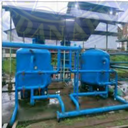
Gambar 3.34 Sand Tank
