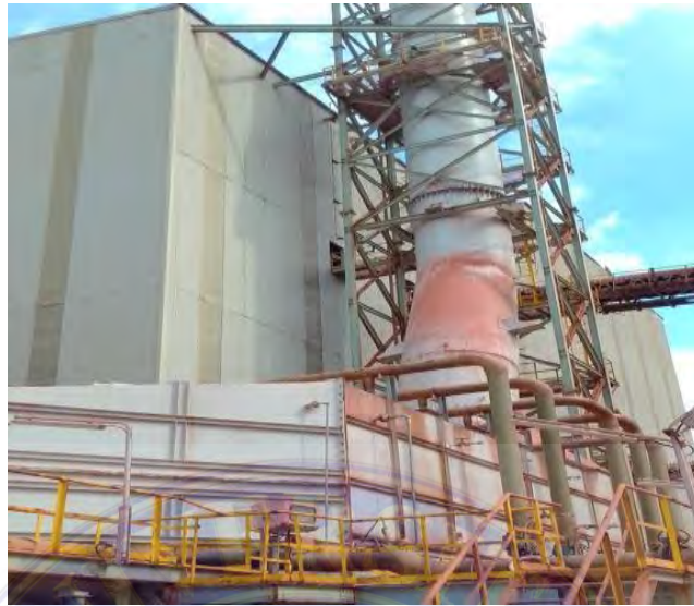
Gambar 3.12 Tail Gas Scrubber (81-D-312)
