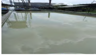
Gambar 3.53 Water Basin (Bak Sedimentasi)
