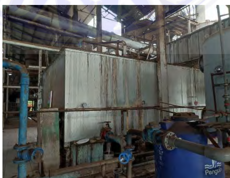
Gambar 3.27 Feed Tank
