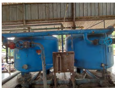
Gambar 3.25 Sand Filter
