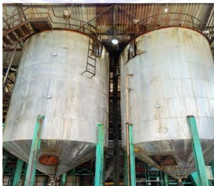
Gambar 3.9 Continuous Settling Tank (CST)
