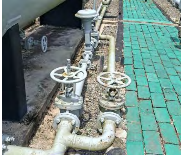
Gambar 3.12 Liquid Control Valve (LVC)
