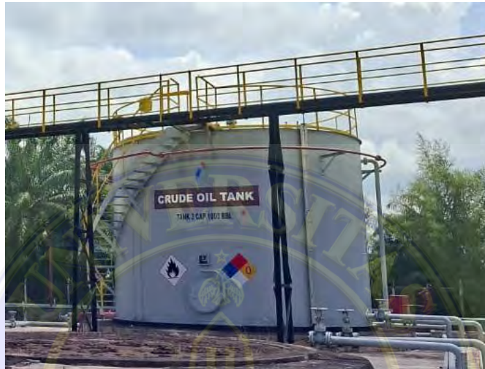
Gambar 3.14 Crude Oil Tank
