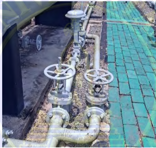
Gambar 3. 12 Liquid control valve
