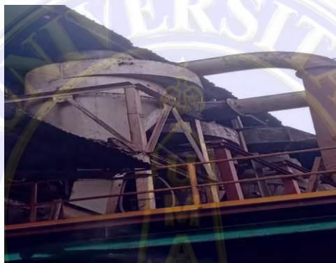
Gambar 3.36. Fibre Cyclone
