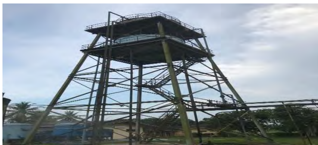
Gambar 3.54. Water Tower Tank
