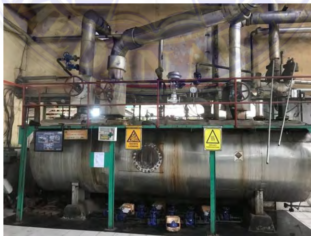
Gambar 3.58. BPV( Back Pressure Vessel )
