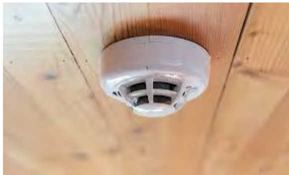
Gambar 2. 14 Fire Alarm & Smoke Detector Protection
