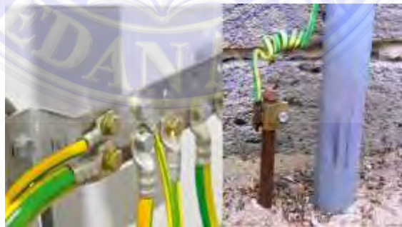
Gambar 2. 7 Grounding System
