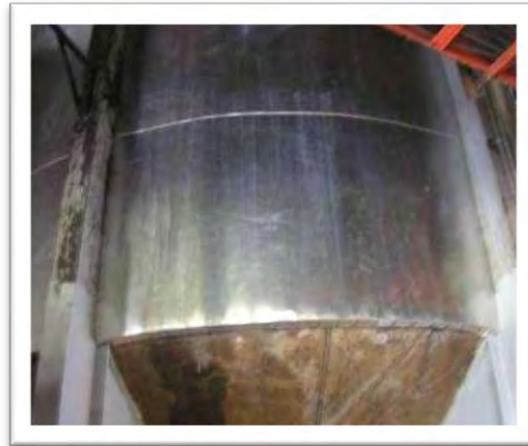
Gambar 3. 33 Clarifier Tank
