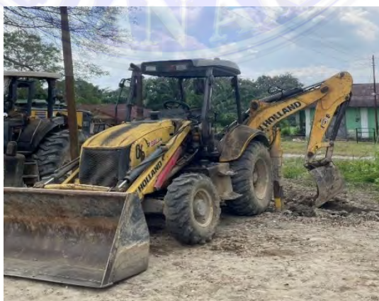
Gambar 3. 1. Backhoe Loader New Holland B90B
