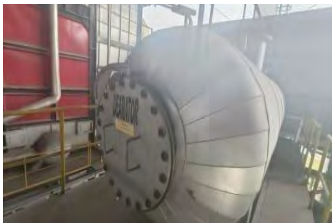
Gambar 3. 43 Dearator Tank
