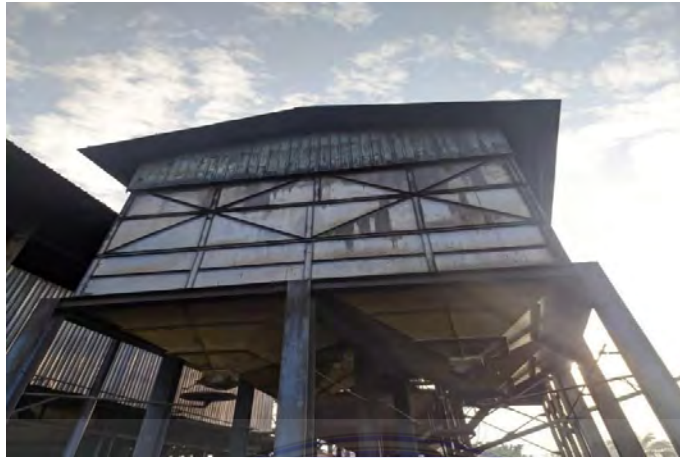
Gambar 3. 31 . Kernel Bunker
