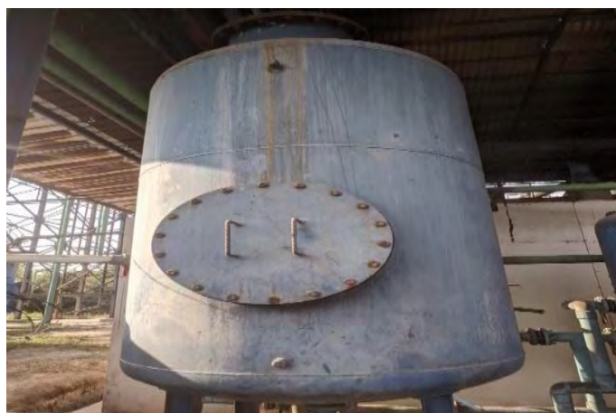
Gambar 3. 40 Softener Tank
