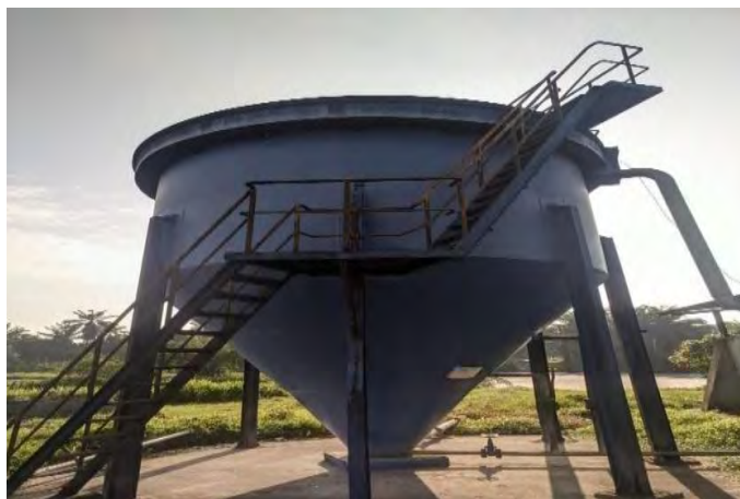
Gambar 3. 36 Clarifier Tank
