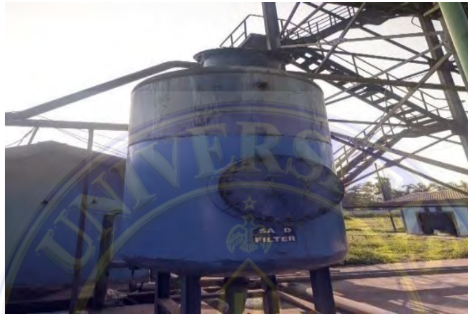
Gambar 3. 38 Sand FilteWater Tank II
