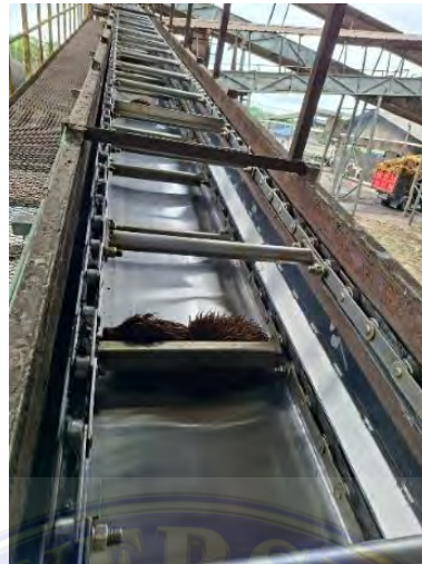
Gambar 3.25 Empty Bunch Conveyor
