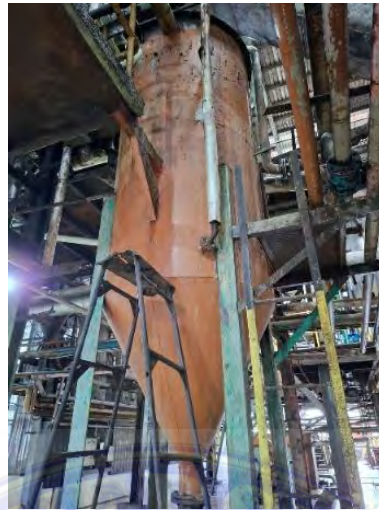
Gambar 3.32 Sand Trap Tank
