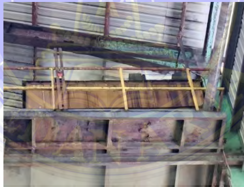
Gambar 3.45 Feeding Separator Tank
