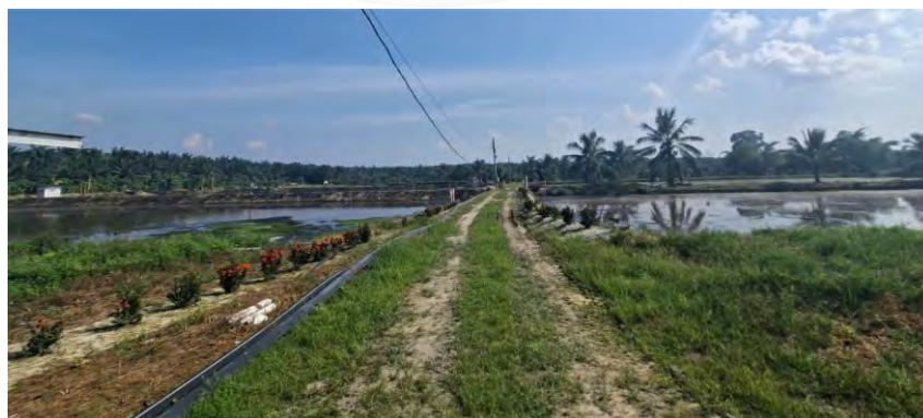
Gambar 3.73 Anaerobic & Aerobic Pond
