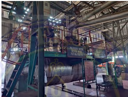
Gambar 3.31 Back Pressure Vessel (BPV)
