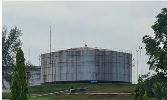
Gambar 3.31 Main Storage Tank ( Tangki Timbun Utama )
