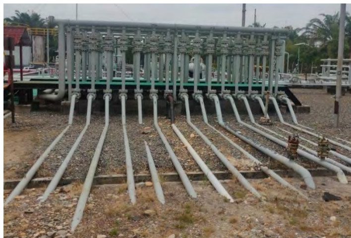
Gambar 3.8 Manifold
