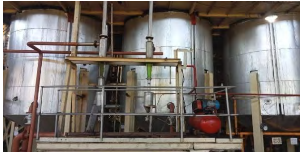
Gambar 3. 19 Sand Trap Tank
