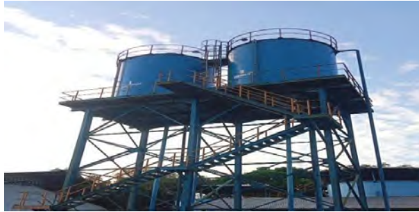
Gambar 3. 55 Water Tower Tank
