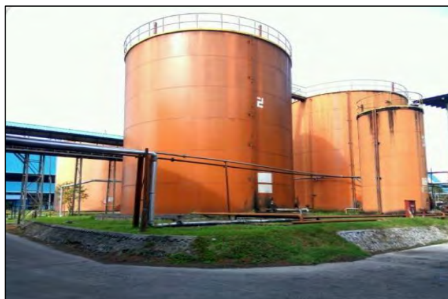
Gambar 3. 23 Oil Storage Tank
