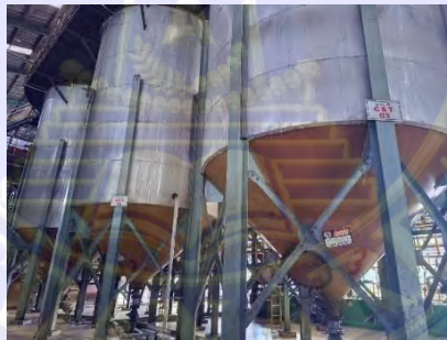
Gambar 3.35 Continuous Settling Tank (CST)
