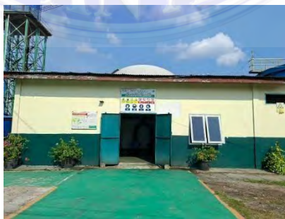
Gambar 3.67 Water Treatment Plant
