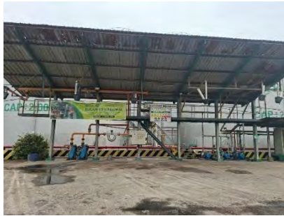
Gambar 3.40 CPO Despatch Area
