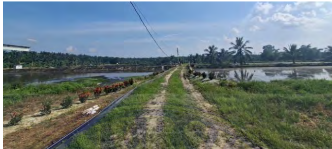
Gambar 3.74 Anaerobic & Aerobic Pond
