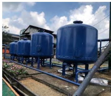
Gambar 3.71 Sand Filter
