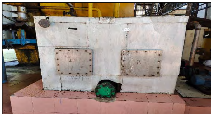
Gambar 3 17 Crude Oil Tank
