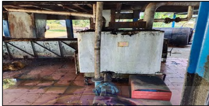
Gambar 3 13 Crude Oil Tank 1
