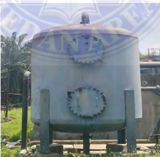
Gambar 4.4 Sand Filter
