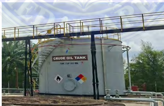
Gambar 3. 14 Crude Oil Tank
