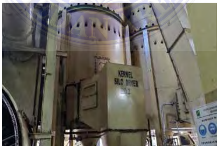
Gambar 3.48 Kernel Silo Dryer
