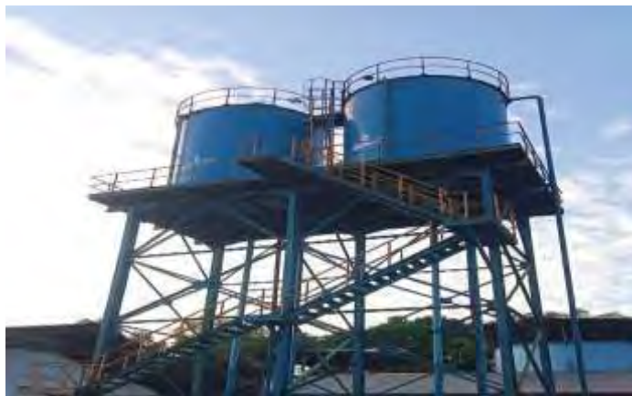
Gambar 3.55 Water Tower Tank
