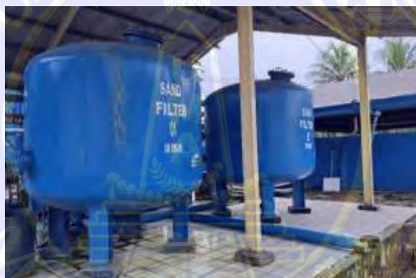
Gambar 3.54 Sand Filter
